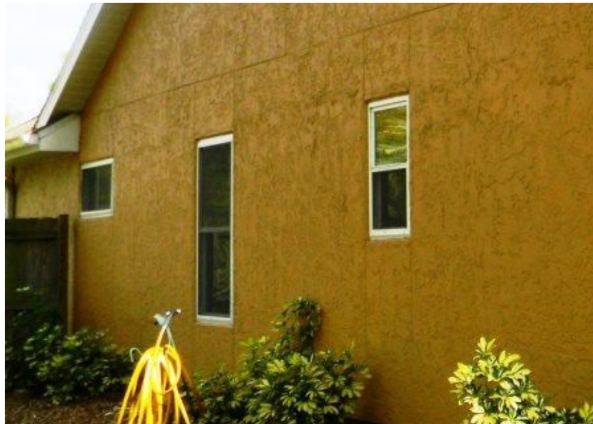
FRAME CONSTRUCTION/ STUCCO ON FRAME
