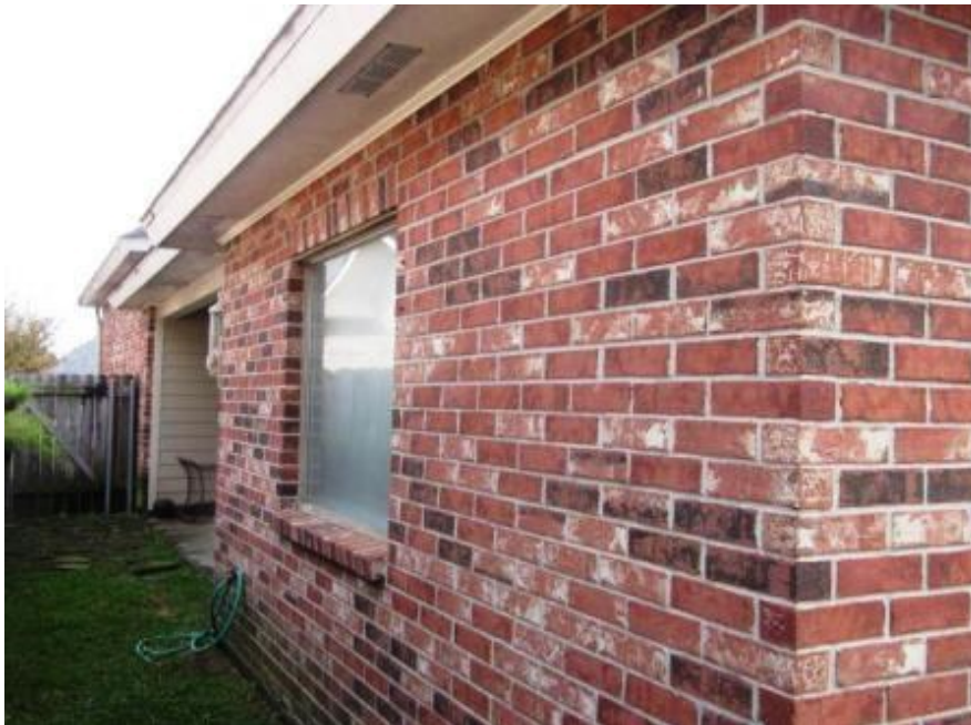
MASONRY VENEER (or BRICK VENEER)
