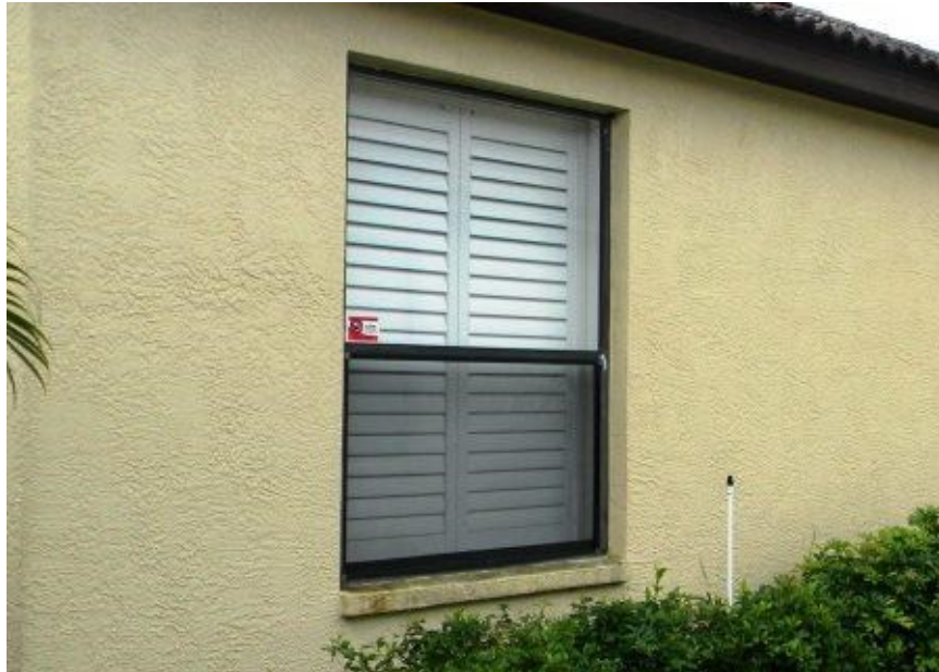
MASONRY CONSTRUCTION/ STUCCO ON MASONRY
